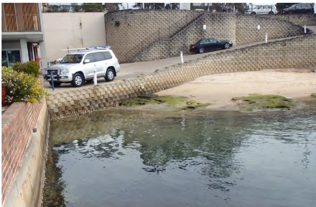
Figure 2-4. Existing stormwater drainage outlet
