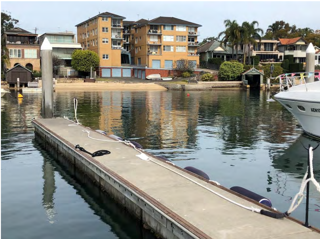
Site Photo at Location #4 (25/7/19)
