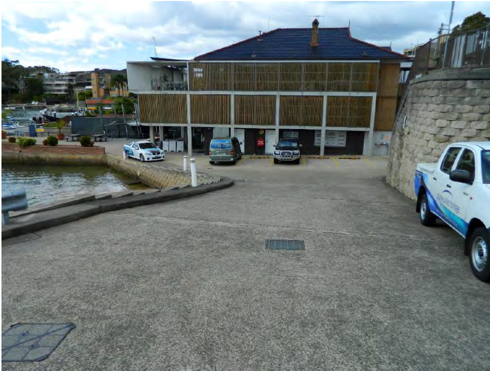
Figure 2-5. Existing stormwater drainage grates
